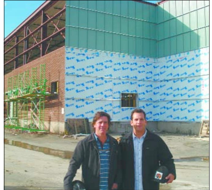
Photos courtesy of Rooflifters
